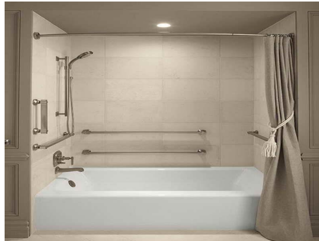
Figure 4 Grab Bars in the Bathtub which is necessary to be added by the Escala Hotel photo adapted from: Pinterest.ph
