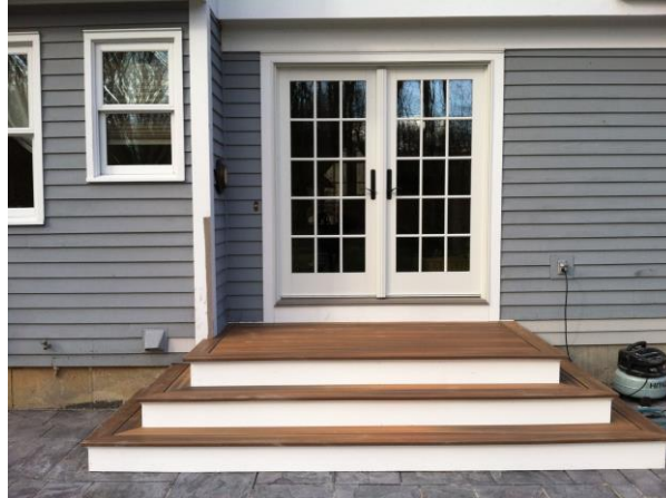
Figure 6: Step Transition in stairs with contrasting color will indicate of the steps photo adapted from: pinterest.ph
